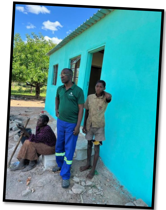
Makuza Completed House Project
